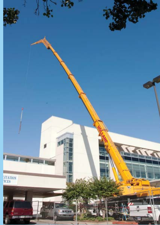
The Foundation provided a significant financial contribution to the construction of two brand new cardiac catheterization labs.
